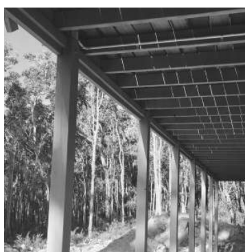
Subfloors and decking posts
