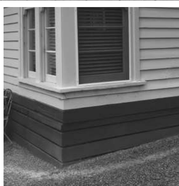
Base boards, retaining walls, fences, exposed rafters
